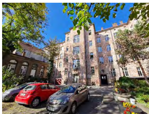
Fig. 11. View of the rear façade of the building of the 20th Secondary School from the south-east side, September 2022.
