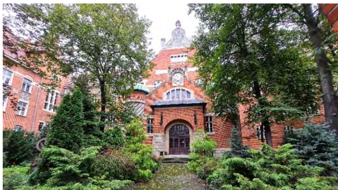
Fig. 25 View of the entrance area to the building of the Mechanical Technical School No. 15 from the west, September 2022.
