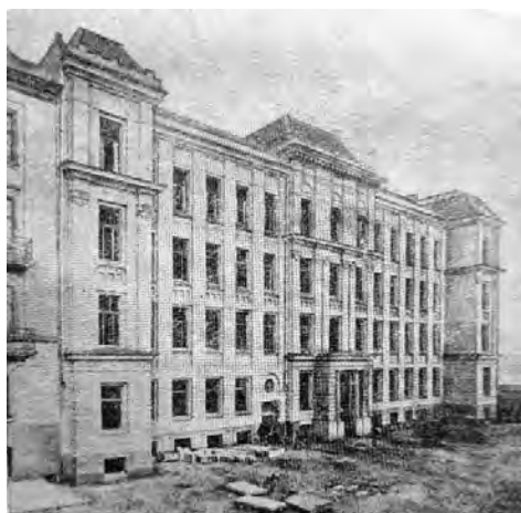
Fig. 7. Design of the front elevation of the building of the 20th Secondary School in Krakow by Jan Zawiejski Dig [19]
