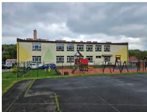
Fig. 2. Primary School in Bezmiechowa Dolna
